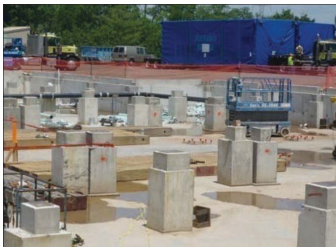
Modular site unique foundation and piers.
