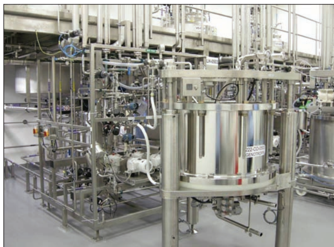
Downstream processing area – chromatography skid and column.
