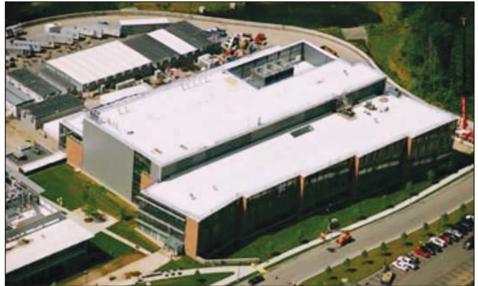
Aerial view of Project Atlas with trailers.
