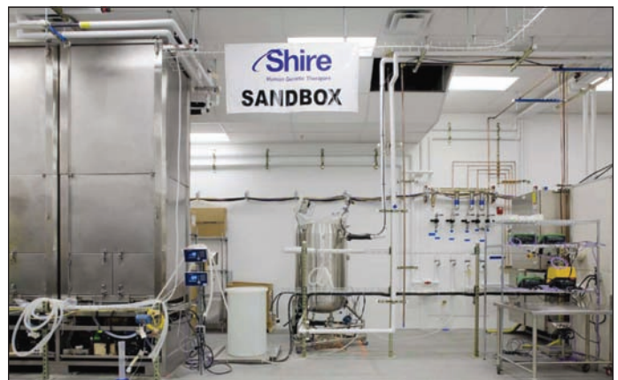
A full working mock-up of the sterile train located offsite.
