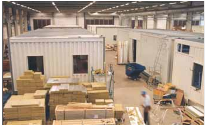
Facility modules built in a workshop environment.
