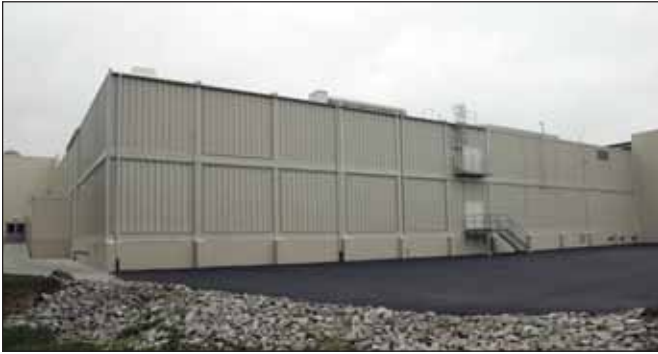
Rear view of the modular manufacturing area.
